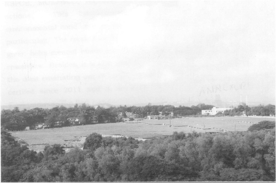
Solar Power Plant at NMPA
