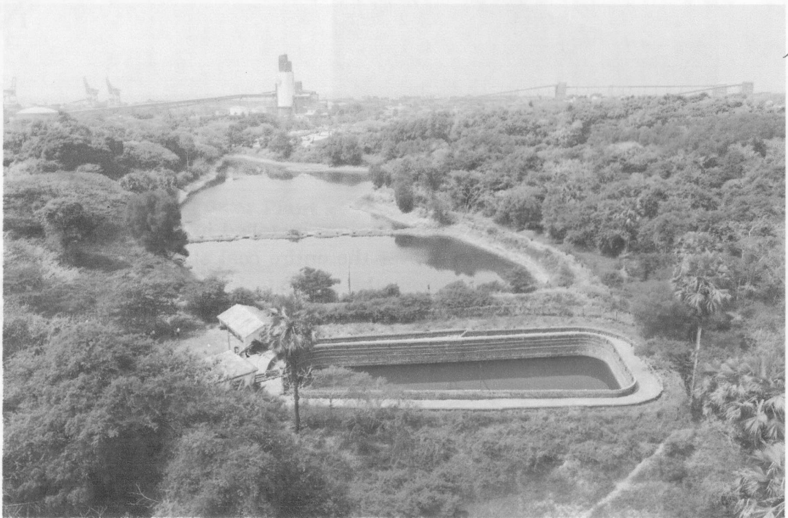
Rain Water Harvesting Near Thimppaiah Well
