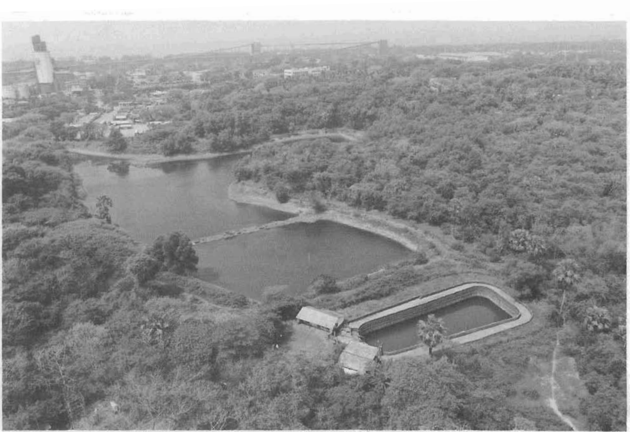
Rain Water Harvesting At Port Estate
