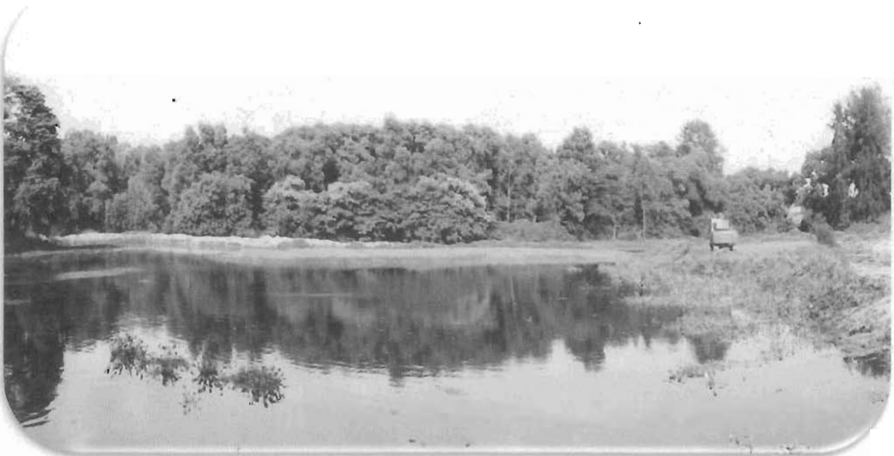
Rain water harvesting at Railway Marshalling Yard
